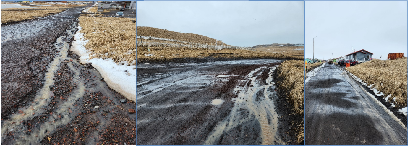
Bartlett Blvd Drainage Documentation
